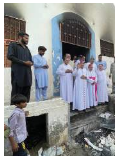
Archbishop surveys damage of church after attacks in Jaranwala.
